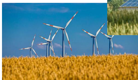
Figure 1: Wind energy. Source: Al3xanderD [1]
