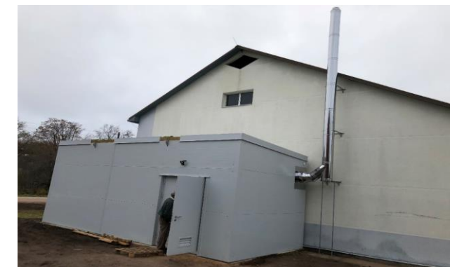
Abb. 22: Heizcontainer, eigenes Foto: V. Kirsanovs [6]
