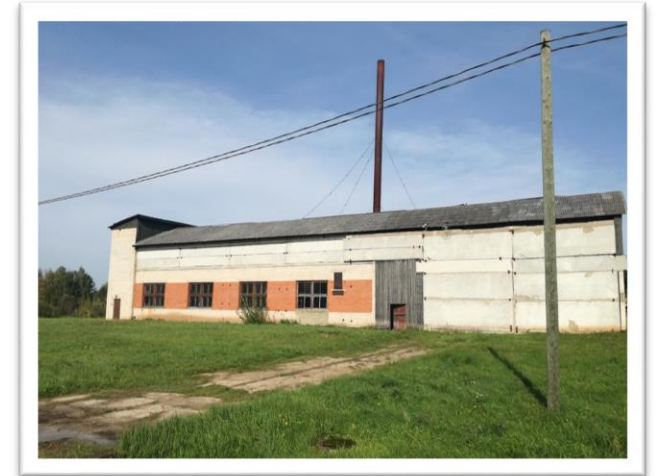
Abb. 21: Heizhaus in Belava, eigenes Foto: V. Kirsanovs [6]
