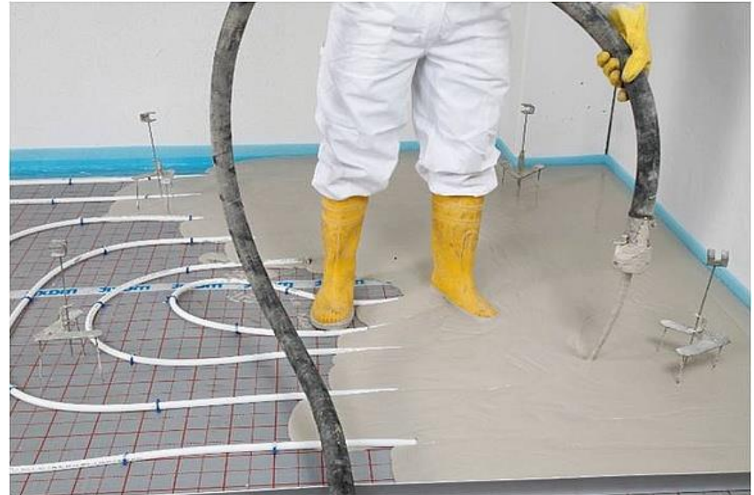
Figure 8: Wet construction, source: www.baulinks.de
